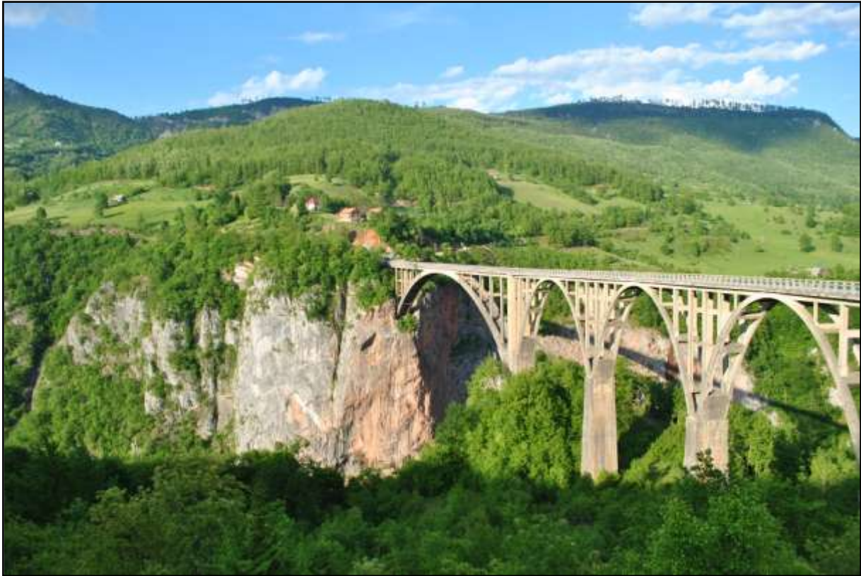
Slika 8 Djurdjevica Tara bridge with the platform
